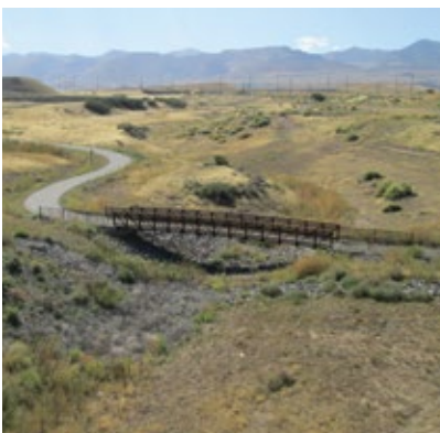
Bingham Creek Bridge
