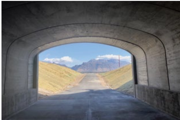
Pedestrian Underpass at 2100 North (UT County)
